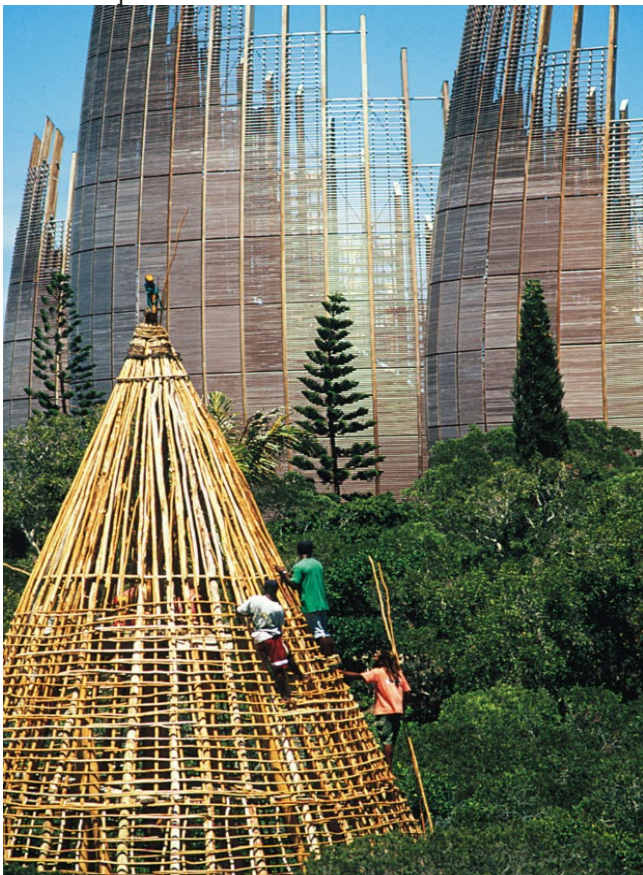
Figure 5b Renzo Piano's Jean-Marie Tjibaou Cultural Center, New Caledonia [b. Kanak roof construction within the site, bottom]
