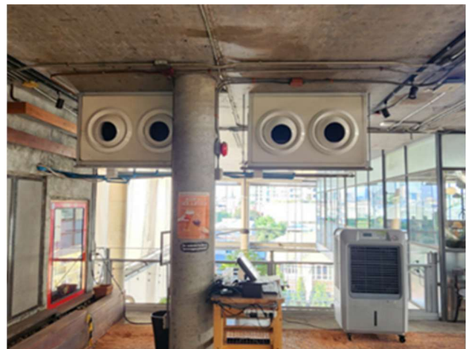
Figure 45 Fourth floor mechanical ventilation system.
