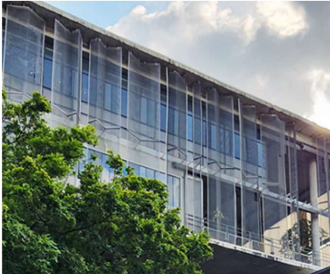
Figure 47 Concrete ledge and expanded metal mesh.
