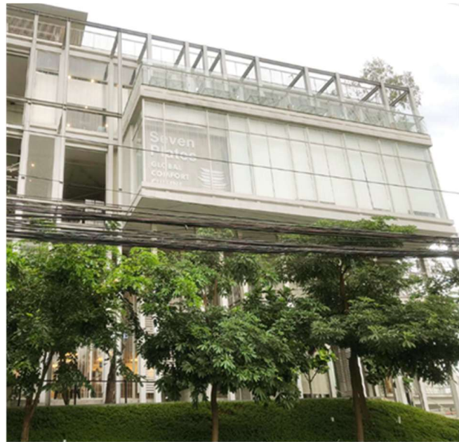
Figure 31 Other landscaping along building perimeter.
