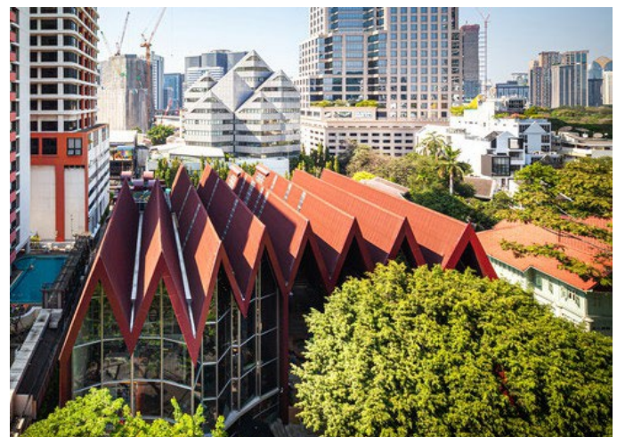
Figure 18 An upper view of the building showing the "M-Shape roof structure"
