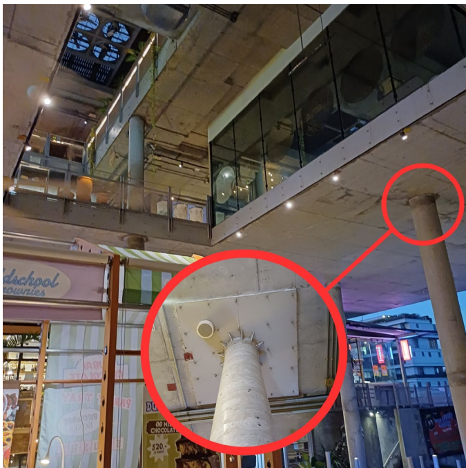
Figure 17 The use of flat slab columns.
